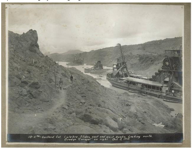
The Panama Canal is widely regarded as one of the 20<sup>th</sup> Century's engineering marvels and the Renfrew-built dredger, the *Corozal*, was instrumental in constructing what is often seen as one of its toughest and most dangerous sections.
