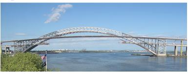
When the bridge was built in 1931 and until recent years the air draft was sufficient for most ships to be able to reach marine terminals in Elizabeth and Newark, New Jersey. But with the size of today's large container vessels, the bridge became an obstacle and without a drastic measure such as "raising the roadway", the Port would lose valuable business
